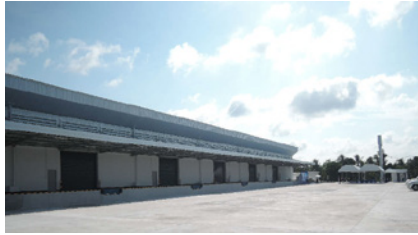
First truck loading dock
