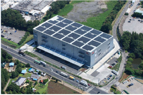
Solar panels on the roof of the Noda Yoshiharu Logistics Center
