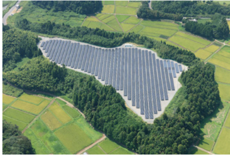
Shibayama solar power plant
