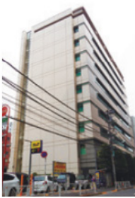
Shibuya Minamiguchi Building Location: Shibuya, Tokyo Site space: 874sqm Floor space: 8,819sqm Completion: Jan. 2000
